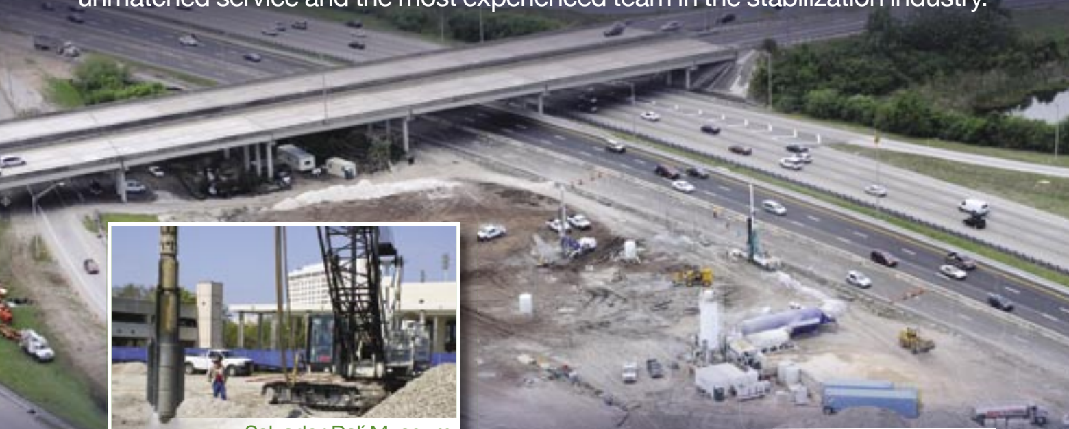
I-4 Interchange Large Scale Sinkhole Stabilization
