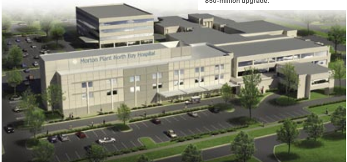
HEALTHY GROWTH Morton Plant North Bay Hospital in New Port Richey is undergoing a $50-million upgrade.
